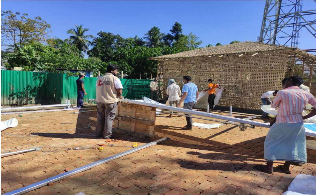
Erection of MSU in Camp 23, Shamlapur
