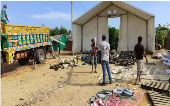
Dismantling of MSU in Camp 2 W
