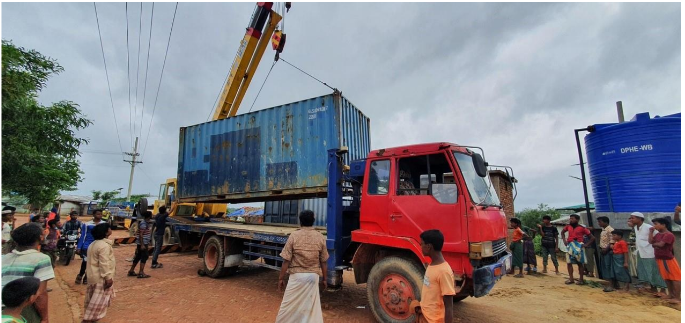
Hope Foundation being supported moving their containers
