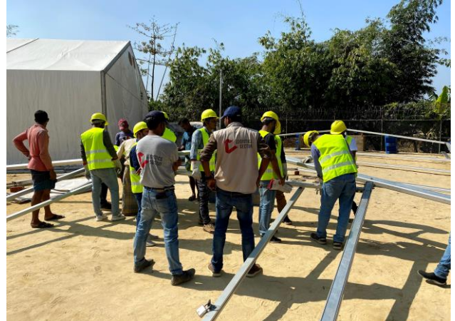
MSU erection training in Balukhali Logistics Hub
