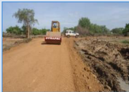
The roller rolling gravel wearing course at IDP site 2—Mingkaman
