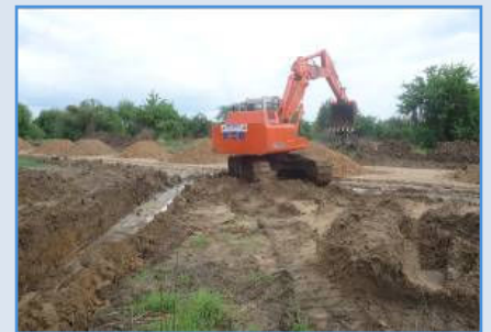
The excavator opening stumps and off shoots in IDP site 1—Mingkaman
