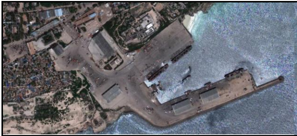
Aerial view of Mogadishu Port, Somalia (Google Earth Image)
