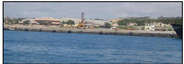
Inner End of North Dock (Port Assessment, Astbury Marine Services)
