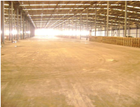
WFP Warehouse in Ganfuda, Benghazi
