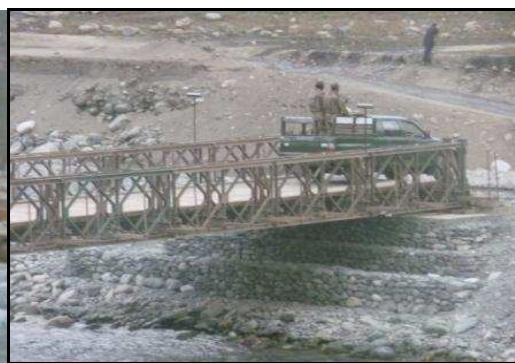
Kalam (KPK) – Newly constructed Bridge
