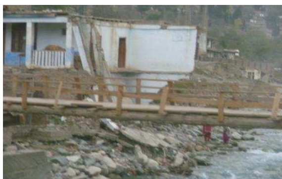
Kalam (KPK) Emergency Log Bridge
