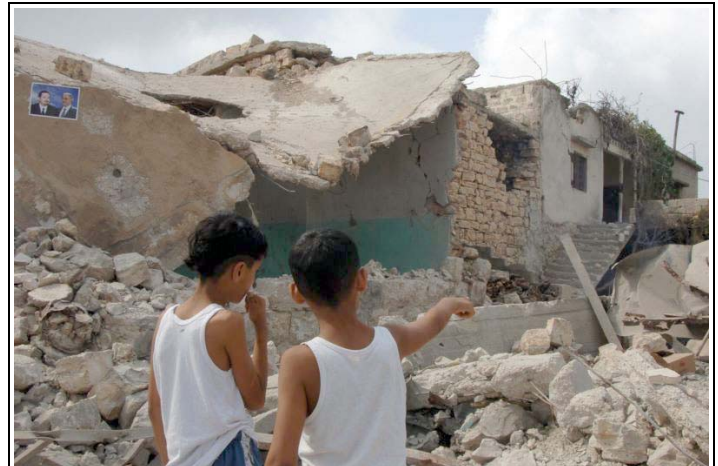
Children in front of rubble in Marwahin south Lebanon
