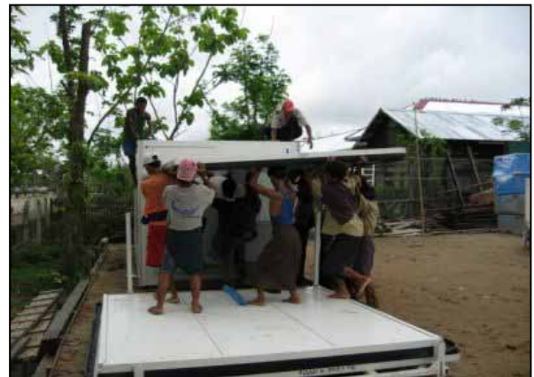
(Assembling of office unit in the Labutta hub)
