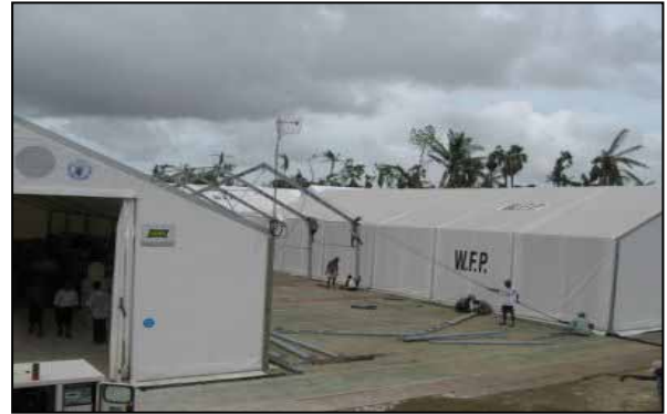
(Erecting storage units and wireless system in the Labutta hub)
